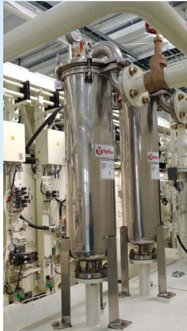
It is suitable for liquid filtration and has a large filtration surface area, which can filter a large amount.]
